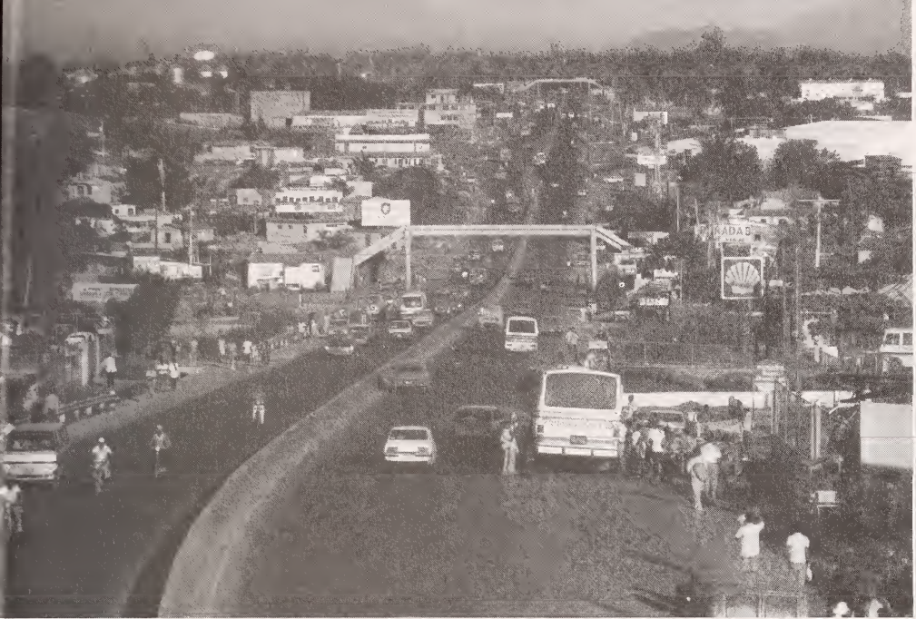
View of the Duarte Highway north of Santo Domingo Courtesy Inter-American Development Bank
