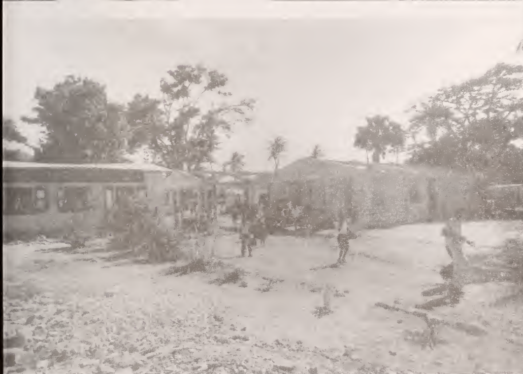
Classroom, University of Haiti, Faculty of Medicine and Pharmacy, Port-au-Prince Partially completed addition to an elementary school Courtesy Inter-American Development Bank
